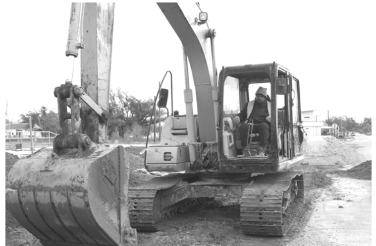
Utility work continues downtown. Photo by Ron Daley
