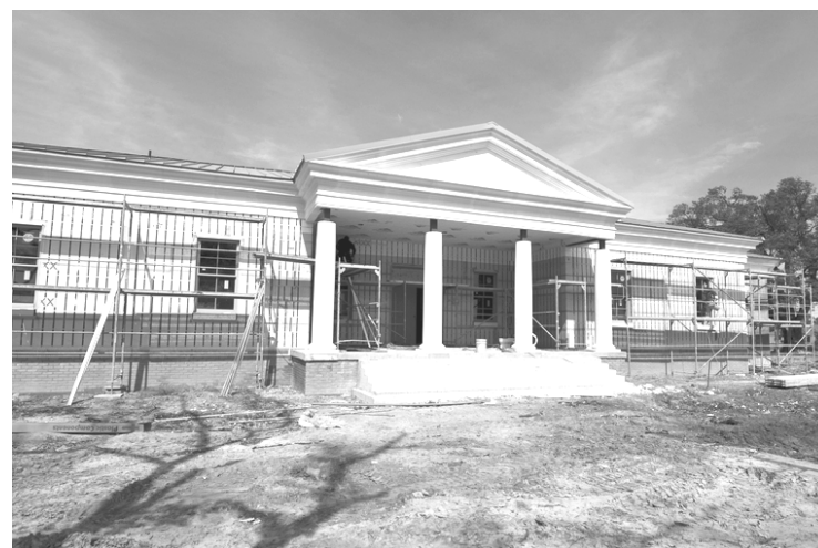
Construction of City Hall is also progressing.
